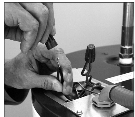
Figure 19 - Connecting the electrical wires.
